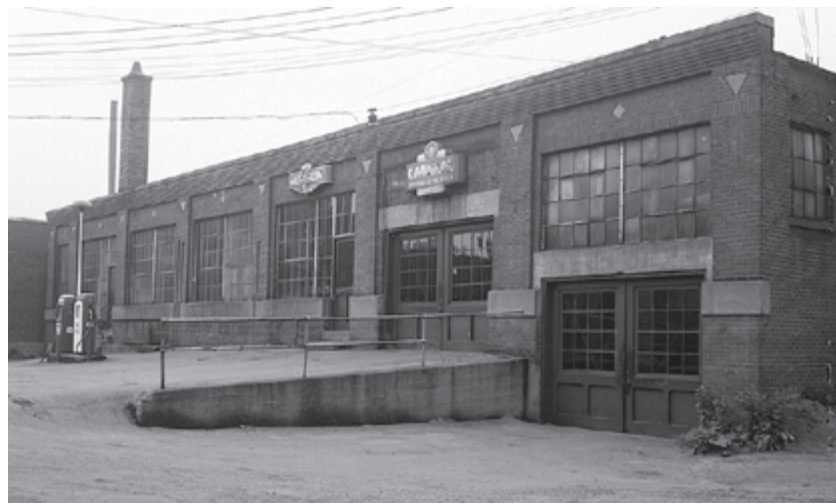
The current location of the Hannah Grimes Center on Roxbury Street.
