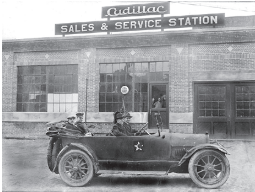
Fairfield's Garage is shown in 1921. Guy Fairfield moved his garage from 58 Beech Street to the old Cheshire House stables at 25 Roxbury Street, Keene in 1913. Fairfield built a two-story building behind Cheshire House not to sell cars, but rather to repair, store, and clean the automobiles of the rich Cheshire House guests. The Cheshire House was renowned for its food and service, and it attracted visitors from all over the world. The Roxbury Street building is now the Blaisdell building.
