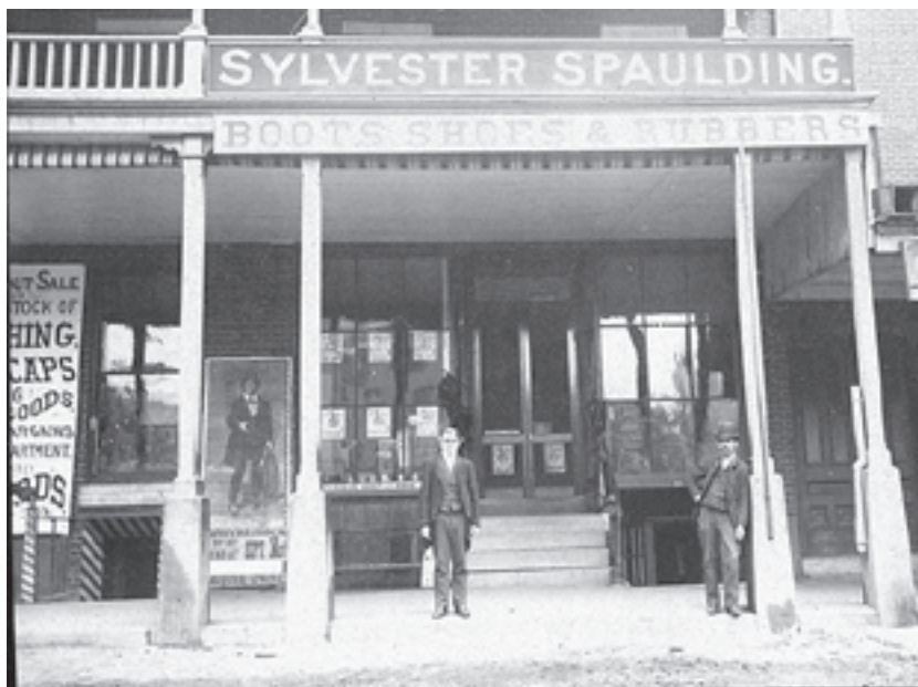
The Sylvester Spaulding Shoe Store and C. Cummings Store on Main Street in Keene were both located in the Cheshire House Block (corner of Main and Roxbury streets) in 1890.
