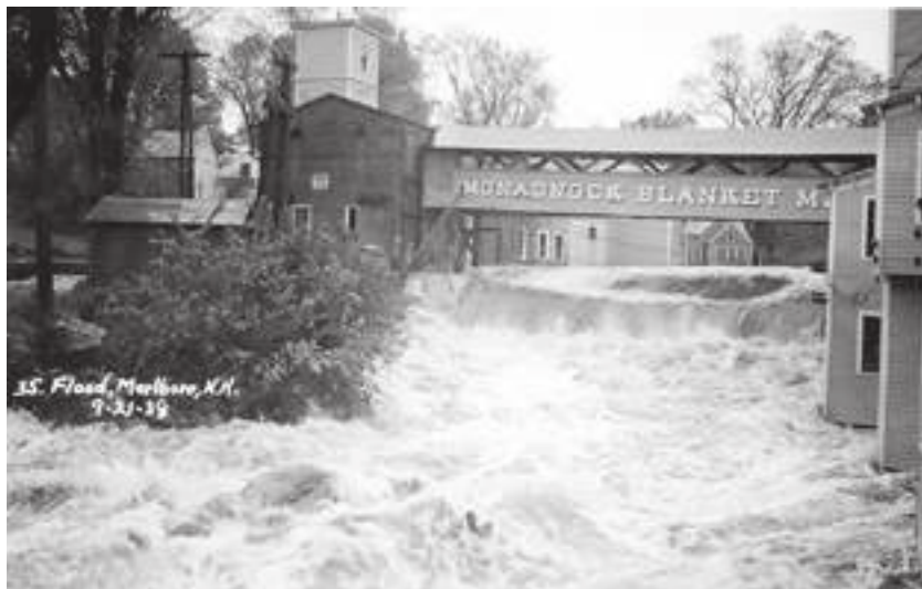
This picture is of the Monadnock Blanket Mill in Marlborough after the 1938 hurricane. The photo shows the company dam and the old mill with the connecting covered walkway to the "new" mill located out of the picture to the right.
