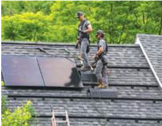
Zach Obuchowski and Camron Tracy of Powers Guaranteed Services on top of a roof working on a solar panel installation.
