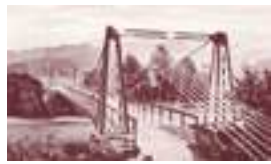
The winner of last week's Mystery Photo was Bernie Cooper of Keene. The bridge, constructed in 1889, connected Chesterfield, NH and Brattleboro, VT.
