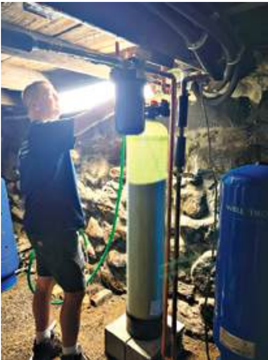
John Wentzel is seen installing a neutralizer filtration system in a house built in the 1700s.
