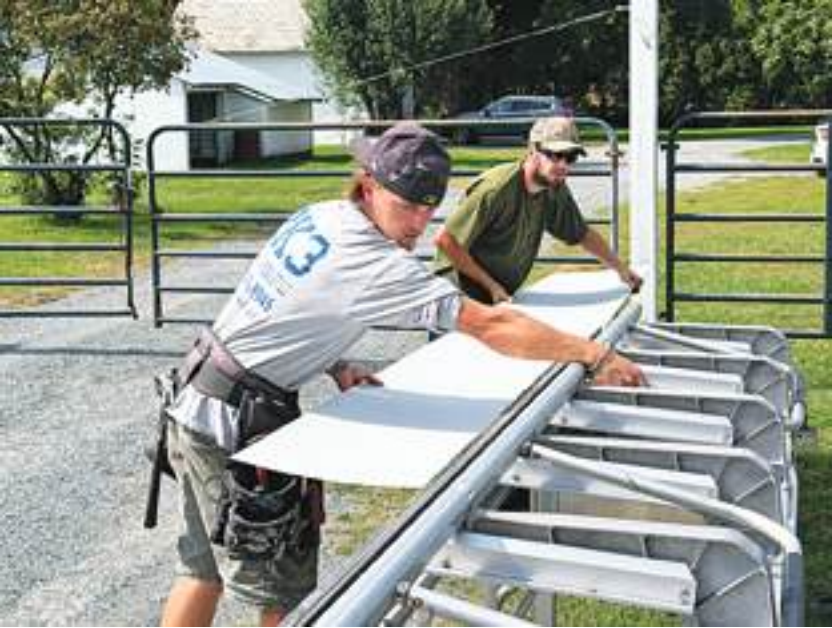
Daniel Tetreault (front) and Patrick Girard of 2K3 Standing Seam Specialist are pictured fabricating a metal starter panel.
