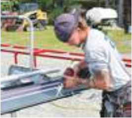
Daniel Tetreault of 2K3 Standing Seam Specialist uses a roll former machine (L), which enables fast and efficient on-site production of standing seam roofing panels. Below, he works on a starter panel.
