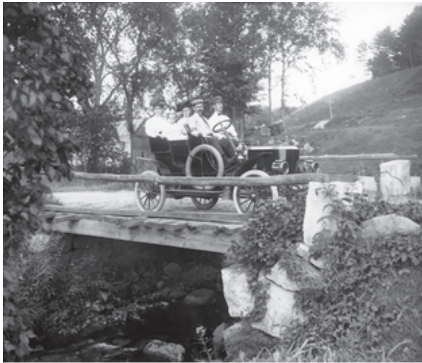
A drive in the country over a wooden bridge, circa 1920.
