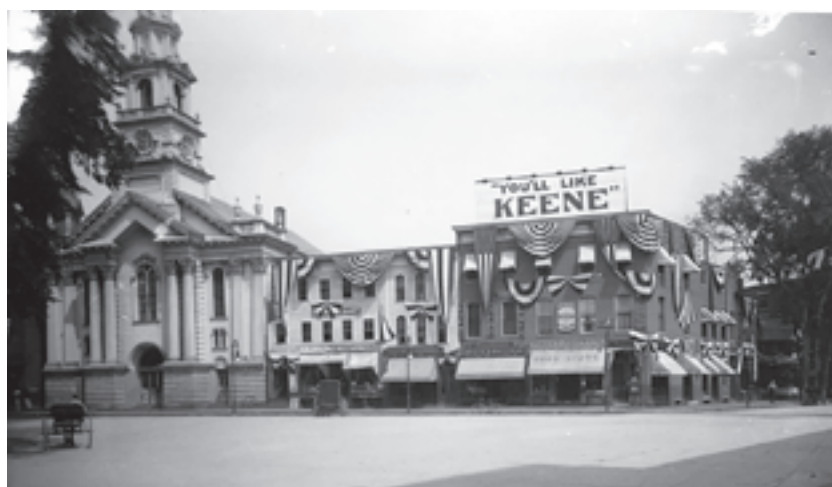
A patriotic bunting is hung with a "You'll like Keene" sign mounted on the roof placed by the Keene Development Company to promote the city as an industrial site, circa 1915. The Congregational Church, B. F. Tyler Confectioner, Central Market, Rossman's Gas & Electric, and Dodge's Pharmacy are pictured in this photo.
